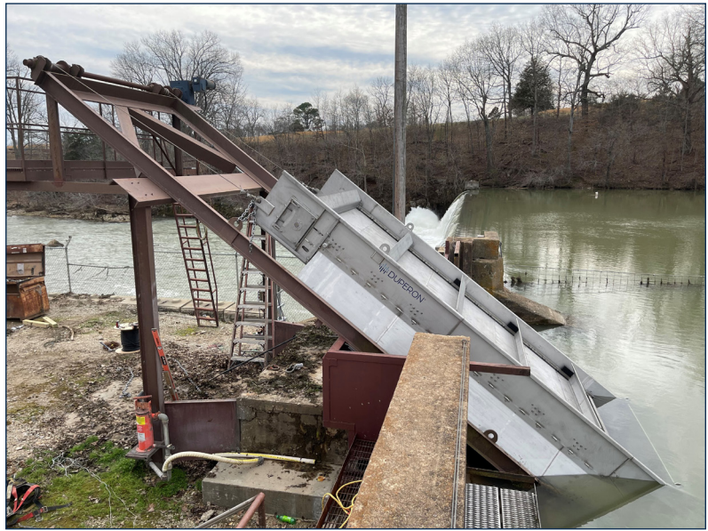
PHOTO 2: New vegetative mechanical screen utilizing existing screen support structure
