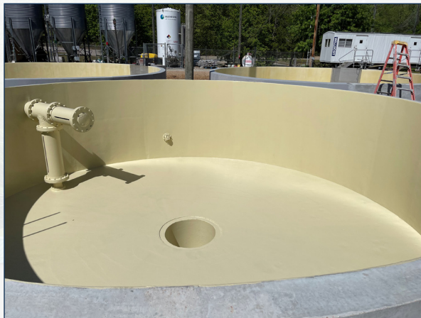
PHOTO 5: High-build epoxy coating to provide smooth surface
