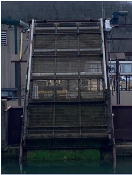
PHOTO 1: Existing chain link vegetative screen
